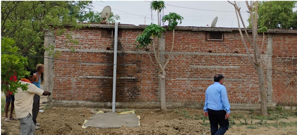
Construction of Perforated Drum-Based Rain Water Harvesting at Pithaipur Hinauti and Katra Narsinghpur under Jal Ganga Samvardhan Abhiyan 2025
